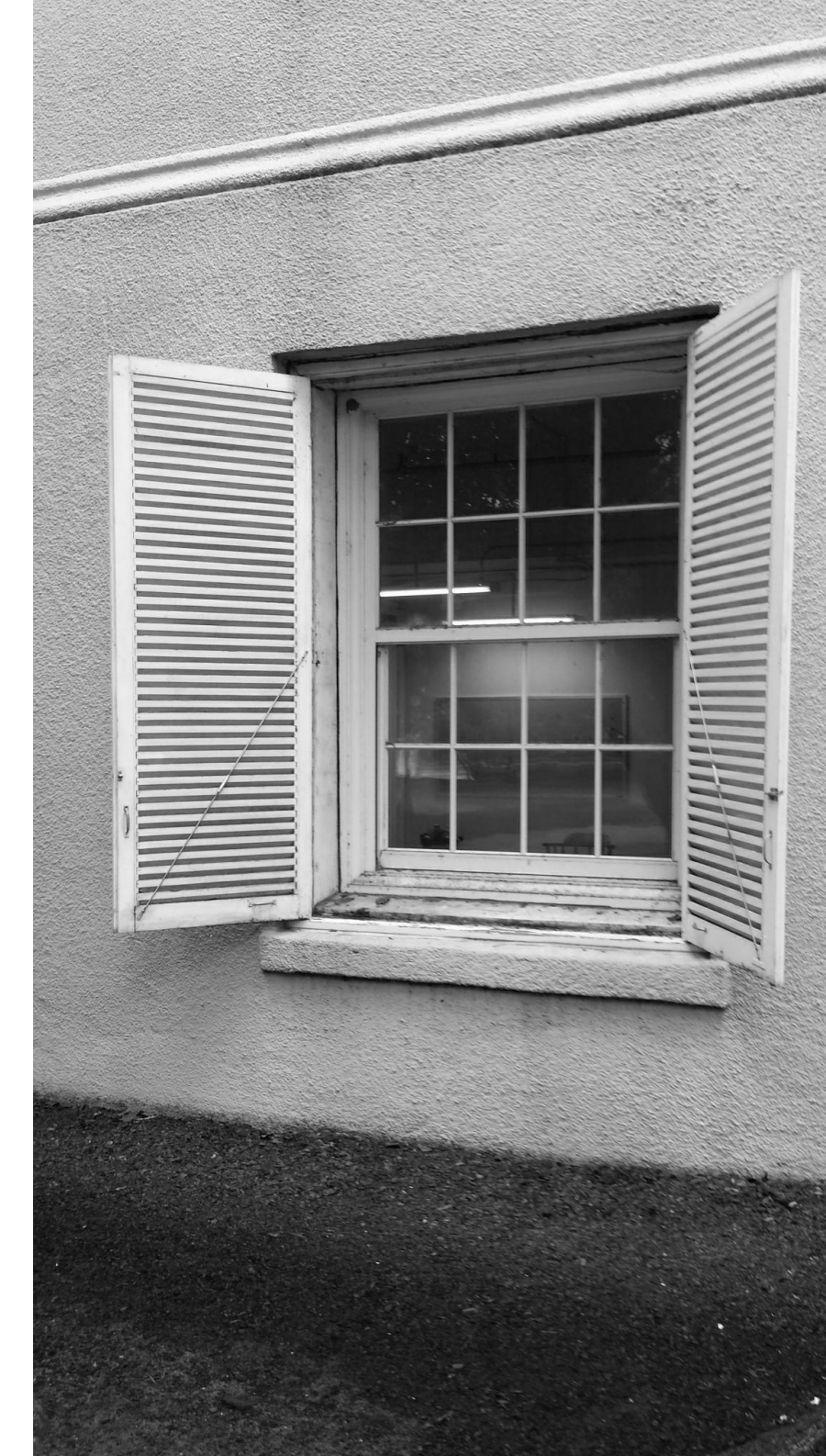
EXISTING OPERABLE SHUTTER ELEVATION
