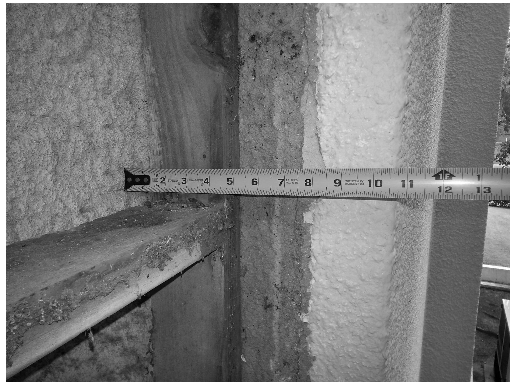
EXISTING WALL SET BACK
